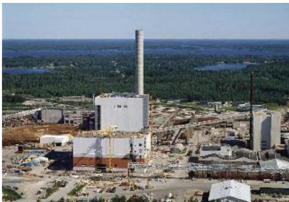
Figure 5 – One of the largest heat and power plants is the Alholmens Kraft facility in Finland, which generates 560 Mega Watts thermal ( $MW_{th}$ ) and 240 Mega Watts electrical ( $MW_e$ )<sup>61</sup> from woody biomass<sup>62</sup>
