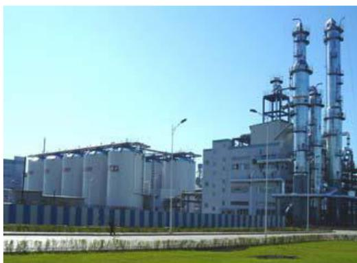
Figure 7 – The world's largest fuel ethanol plant, Jilin, China, processes close to 2 M tonnes of corn per year to produce some 2.3 Ml per day ethanol<sup>73</sup>
