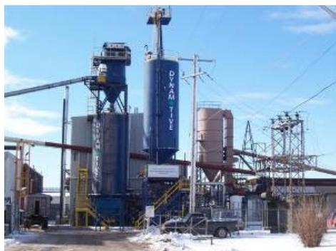
Figure 9 – Dynamotive flash pyrolysis plant in West Lorne Canada<sup>79</sup>
